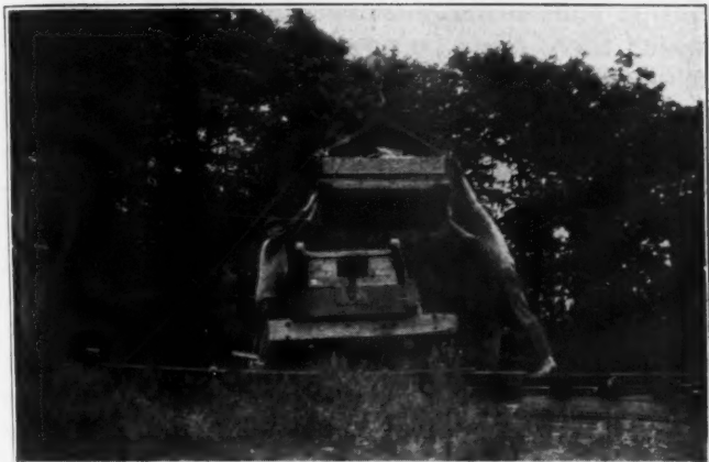
Placing a Skip Load of Waste on the Push Car for Disposal at the Dump
